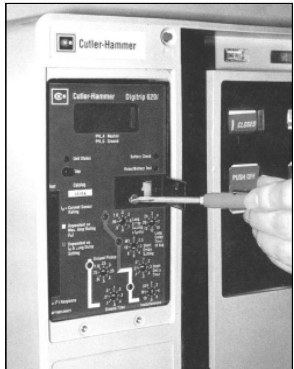
Figure 1.3 Installation of the Rating Plug and Mounting Screw
