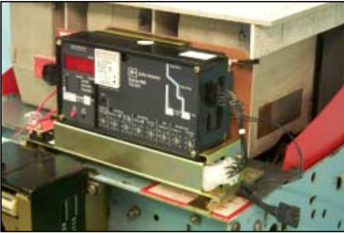
Fig. 50 Overview: Aux. CT Assembly and Trip Unit Installed on the Breaker.
