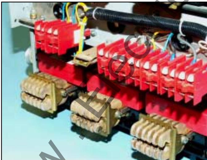
Fig. 9 Finger Clusters Reinstalled on the Load Terminals (Electrically Operated).
