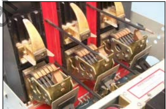
Fig. 2 Hood Assembly, Arc Chutes, Flash Barrier, Interphase Barriers, and Side Barriers Removed from the Breaker.
