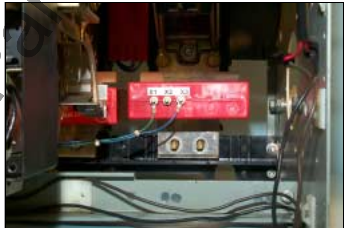
Fig. 10 Sensor Harness Connected to the Sensors.
