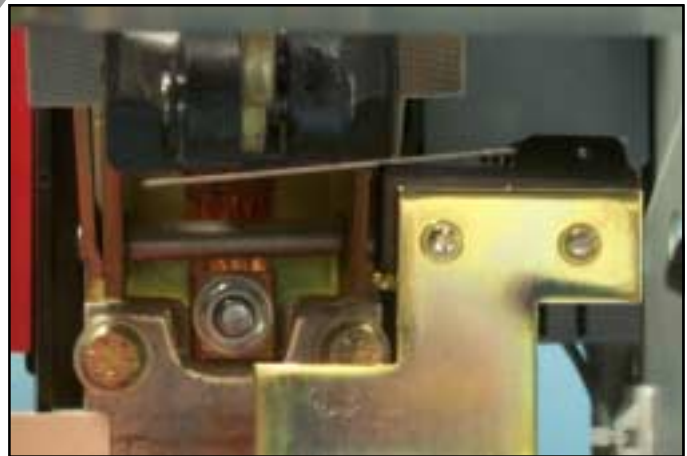
Fig. 28 Correct Engagement of the Auxiliary Switch Arm.
