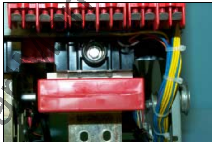
Fig. 7 Sensor and Spacers Installed on a Jumper.
