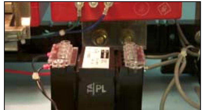
Fig. 24 Finger-Safe Covers Installed on the CPT Module.
