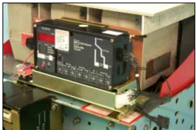
Fig. 58 Rating Plug and Aux. CT Harness Installed.
