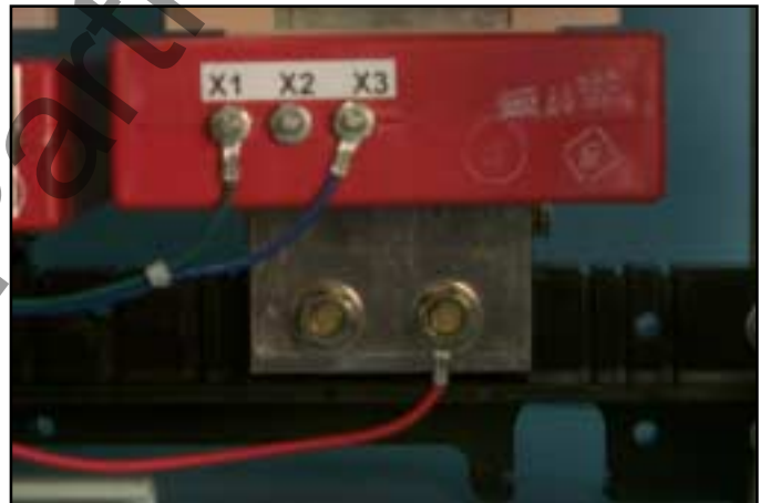
Fig. 16 PT Wires Connected to the Jumper Bolts.
