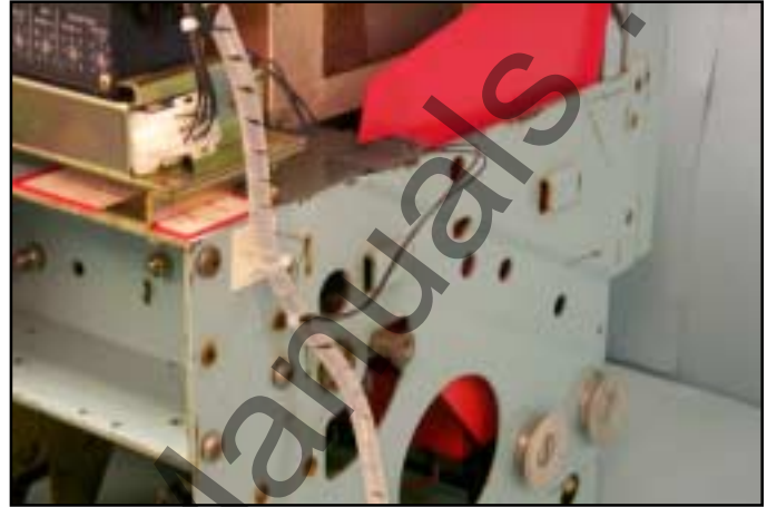
Fig. 63 External Harness Secured to the Side of the Breaker.
