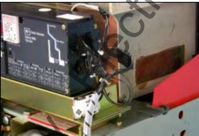
Fig. 62 External Harness Connections at the Trip Unit.
