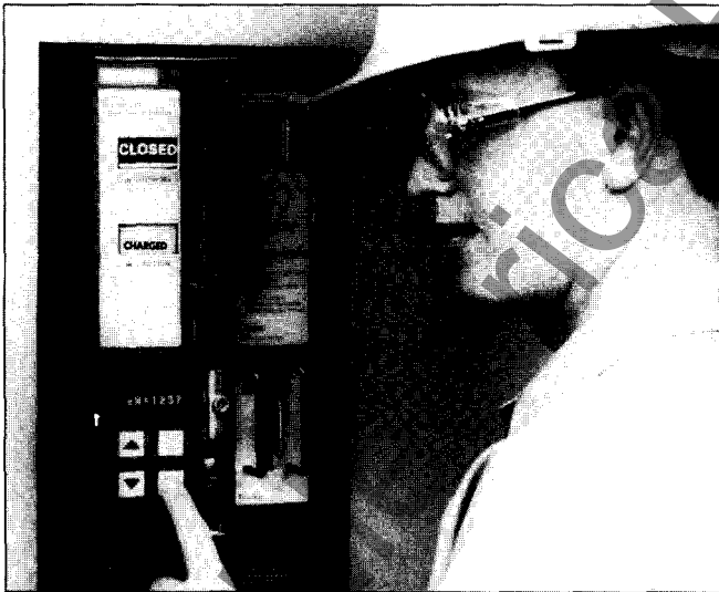
BDU Mounted on Type RL circuit breaker
