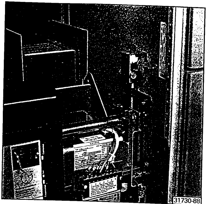
Figure 14. Key Interlock Located in Circuit Breaker Compartment
