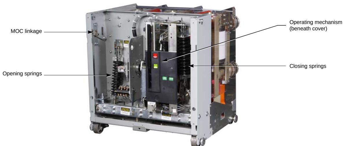
Figure 5: Circuit Breaker—Left Front View with Cover Removed
