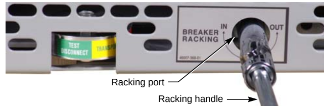
Figure 20: Racking Handle Engaged onto Racking Shaft with Circuit Breaker in the TEST/DISCONNECT Position
