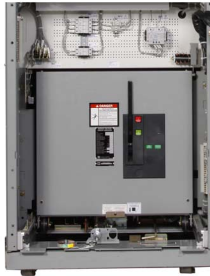
Figure 15: Type VR Circuit Breaker in the TEST/DISCONNECT Position (Lower Compartment)
