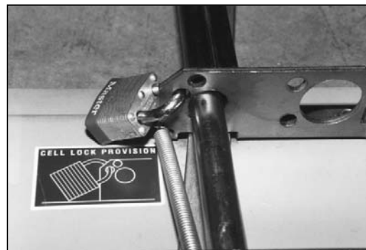
Figure 21: Racking Mechanism Padlock Provision
