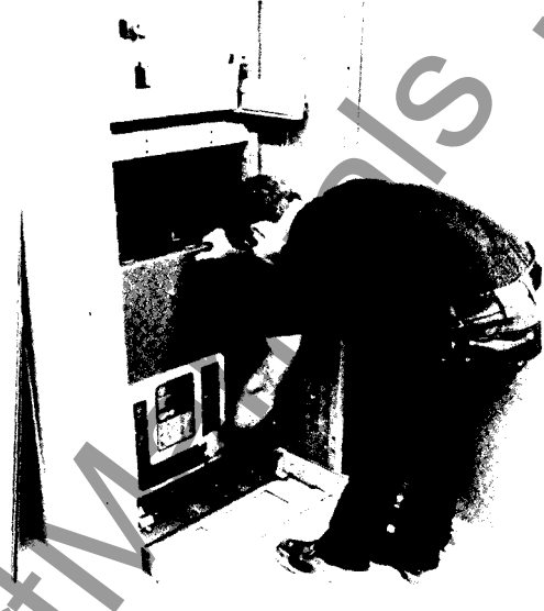
b. Pulling the Breaker Out on the Extension Rails Note That Lift/Pull Handle Must Be Lifted to Pull the Breaker Out
