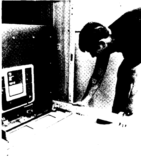
a. Engaging the Extension Rails Before Removing the Breaker
