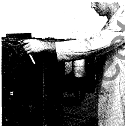
11. Holding The Interrupter Assembly With One Hand, Remove The Last Mounting Bolt Of The Upper Insulator
