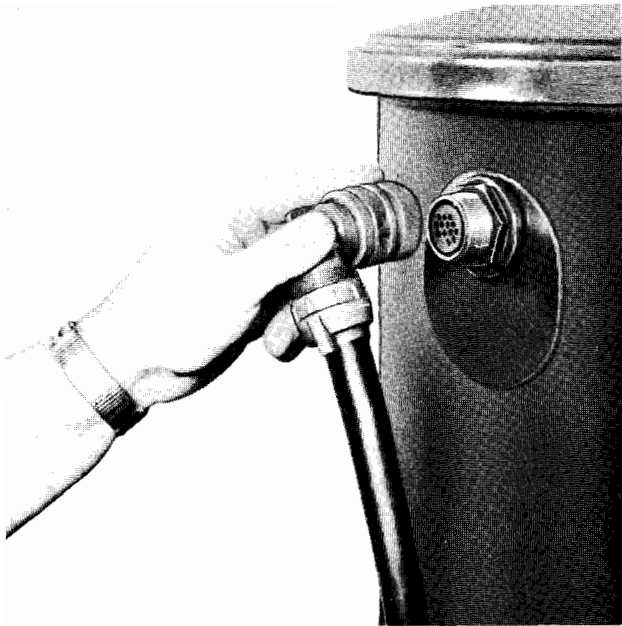
Fig. 11 - Disconnecting Flexible Cable from Regulator Tank
