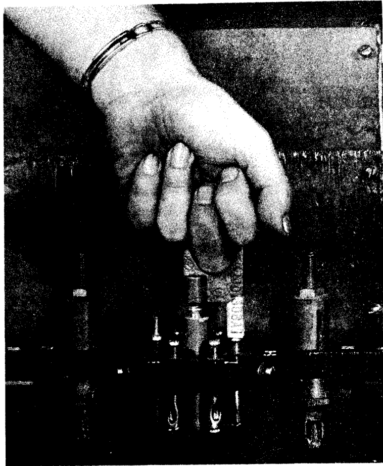
FIG. 17 SETTING TAP SELECTOR SWITCH
