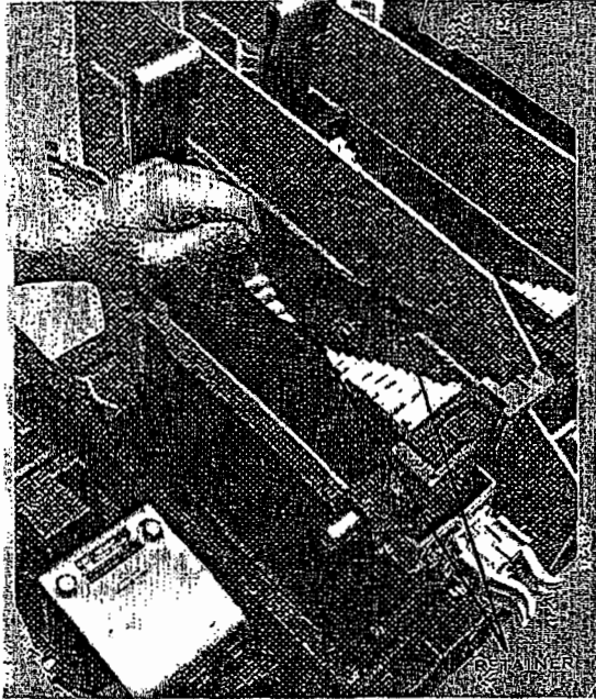
Fig. 23. Removal of arc-barrier retainer
