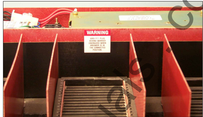
Fig. 24 PT Warning Label Installed on the Front Aux. CT Module Insulation Barrier.
