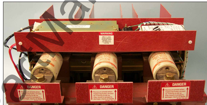
Fig. 25 PT Warning Label Installed on the Rear Aux. CT Module Insulation Barrier.
