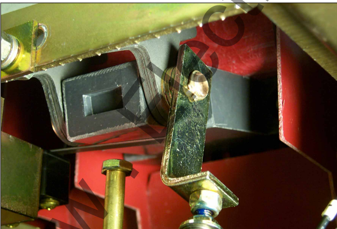
Fig. 38 Reset Assembly Mounting on a LAF-1600 B Breaker.
