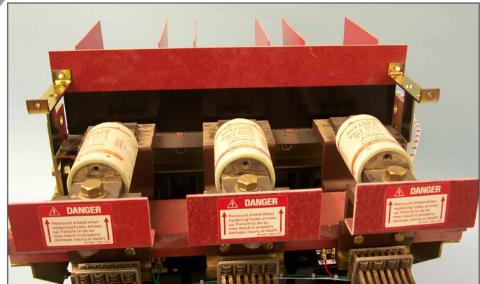
Fig. 12 Front Aux. CT Module Insulation Barrier Installed on the Mounting Brackets.
