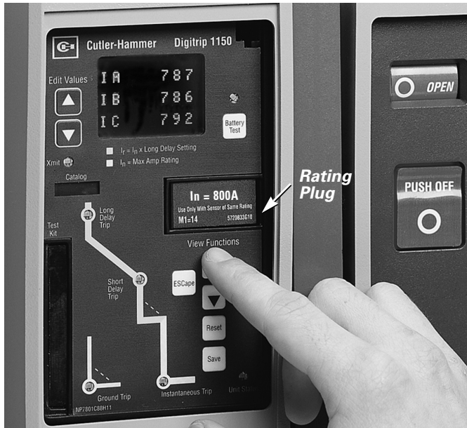
Figure 6-6 Trip Unit Rating Plug Location
