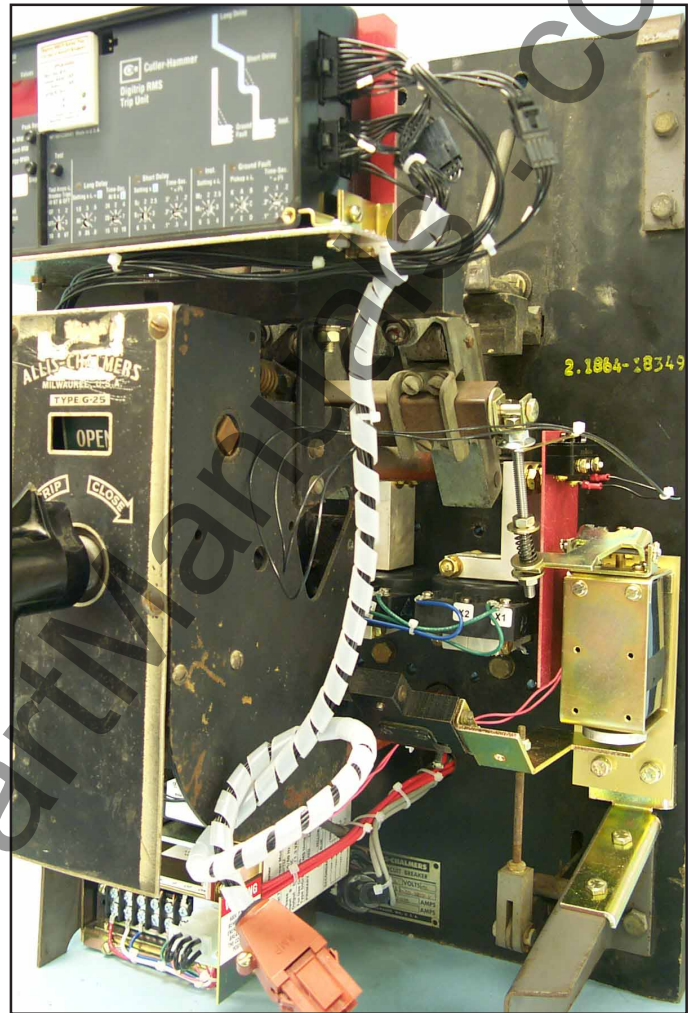
Fig. 64 External Harness Connections at the Trip Unit.
