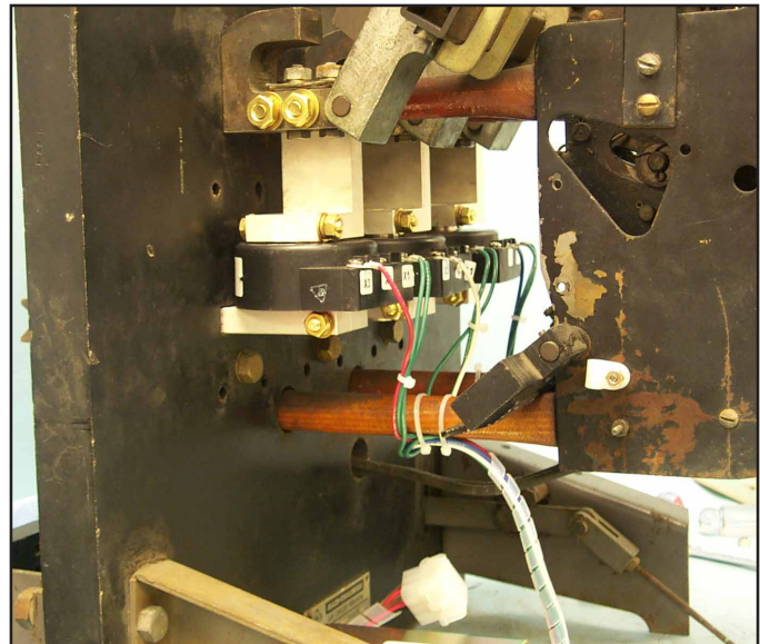
Fig. 13 Sensor Harness Connected to the Sensors.
