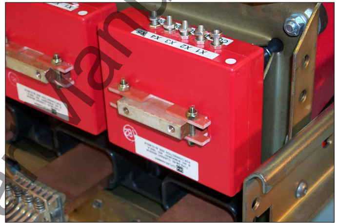
Fig. 6 Correct Positioning of the Sensors and Spacers.
