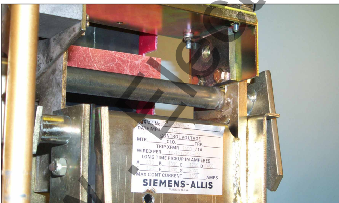
Fig. 19 Correct Orientation of the Bearing Caps and Trip Unit / Aux. CT Module Assembly Mounting Bracket.
