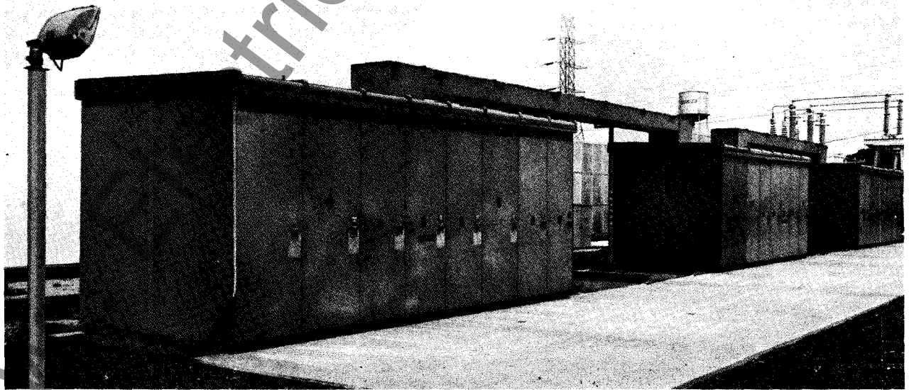
SUBSTATION furnished with General Electric's outdoor metal-clad switchgear.
