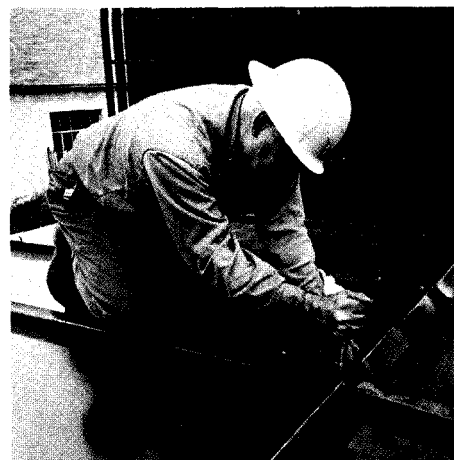
4. VENT CAPS are bolted on roof to form completed weatherproof assembly. Breakers are moved into place.
