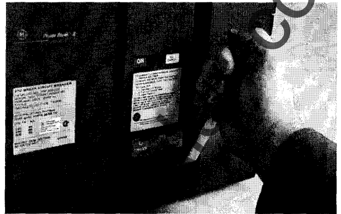
Operation of circuit breaker pump handle
