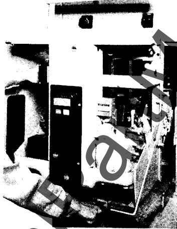
Fig. 33 Drawout Tray In Position To Receive AK-50 Breaker
