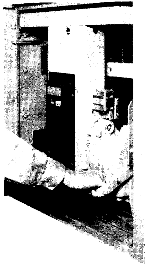
Fig. 38 Racking Handle At End of Fifth Stroke
