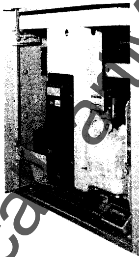
Fig. 39 AK-50 Breaker In "Connected" Position
