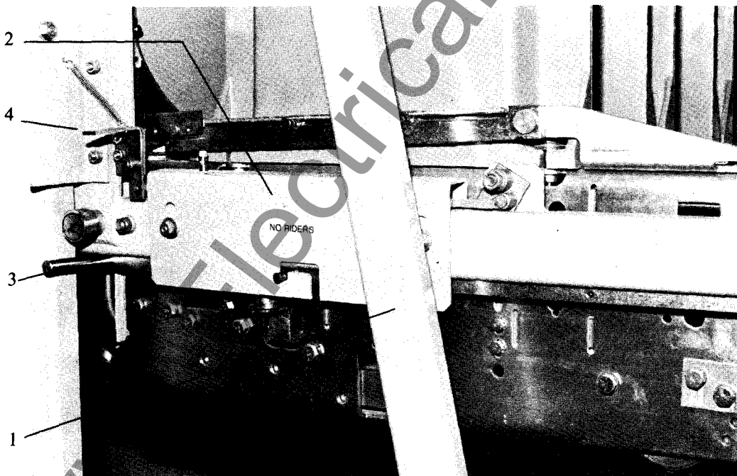
Fig. 38 Lift Truck Connection to Rails
