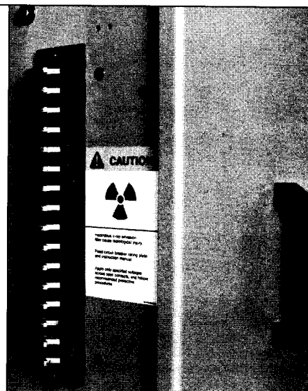
Secondary Disconnects (Cubicle portion on left, Breaker portion on right)
