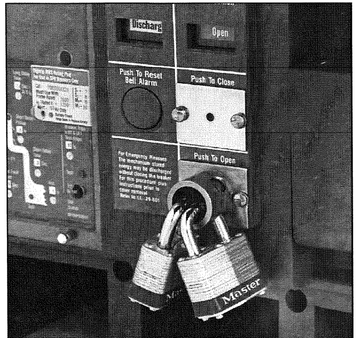
Figure 5-15 PUSH-TO-OPEN Padlockable Kit Installed
