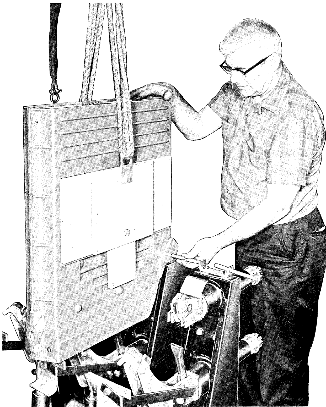
Fig. 2b. Installing Arc Chute of Type 150-DH-P500 Breaker
