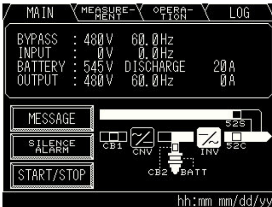
FIGURE 2.7-a Main screen (Battery operation)
