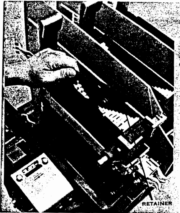
Fig. 23. Removal of arc-barrier retainer
