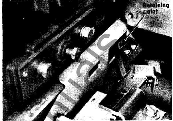
Fig. 35. Closeup of contactor, showing retaining latch.
