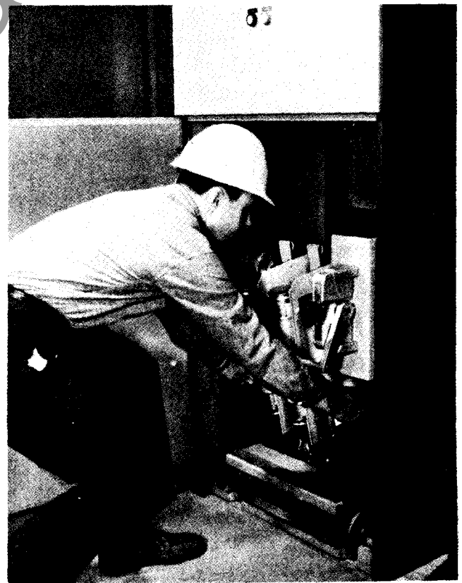
Fig. 81. Push contactor in enclosure by pushing on side frames.
