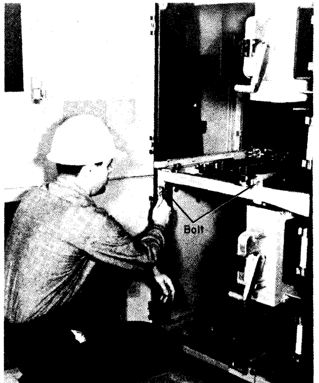
Fig. 50. Removing bolts in track and horizontal barrier assembly in three-high enclosure.
