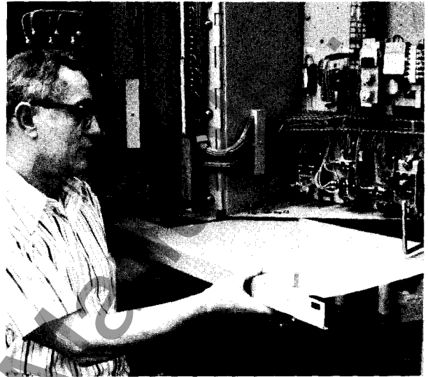
Fig. 29. Horizontal shelf and barrier removal.
