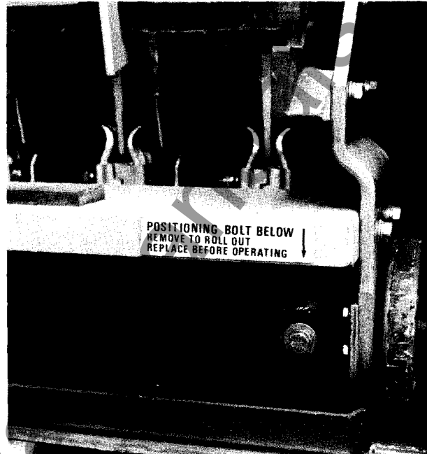
Fig. 25. One-high contactor in enclosure showing positioning bolt that must be removed to roll out contactor.
