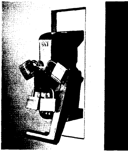
Fig. 8. Limitamp isolator handle padlocking provisions.
