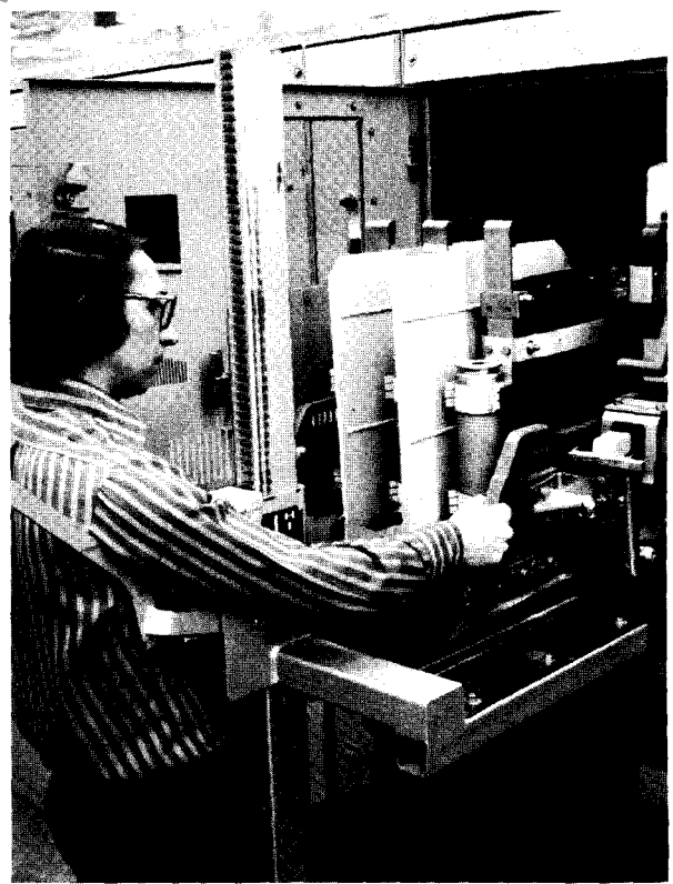
Fig. 36. Removing contactor, using Cat. No. 116C9918G1 lift.
