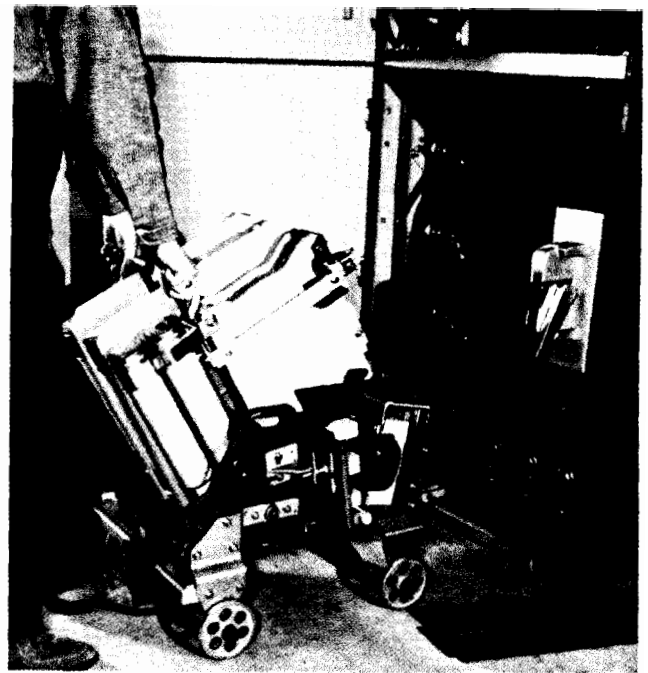
Fig. 92. Swinging high-voltage contactors open for inspection.
