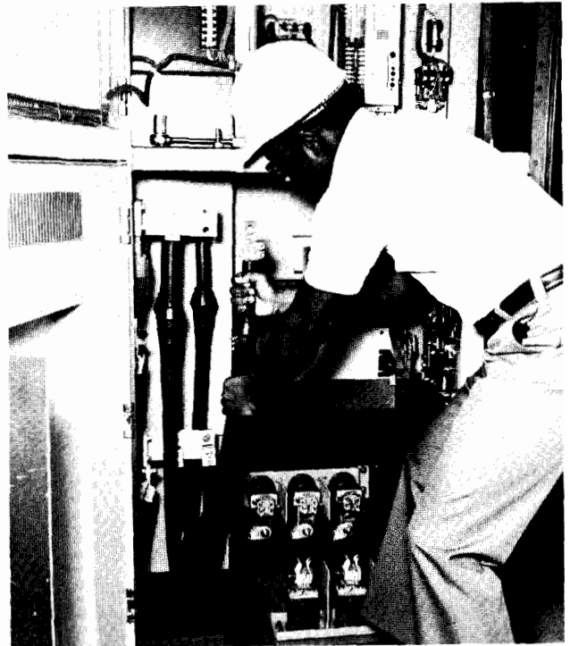
Fig. 65. Extra-width enclosure for motor cable.
