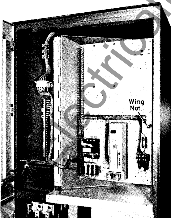
Fig. 80. Wing nut which holds swing base of one-high enclosure.
