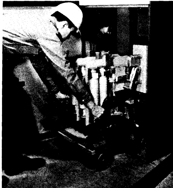
Fig. 26. Roll contactor out of enclosure.
