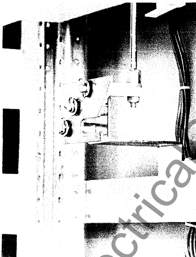
Figure 13. Contactor engagement pawl for mechanical interlock
