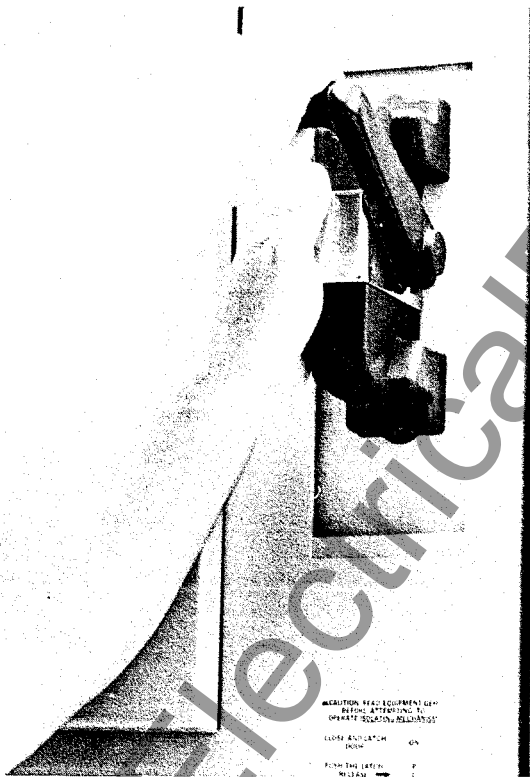
Figure 17. Operate handle by depressing handle latch release with one hand and moving the handle with the other.
