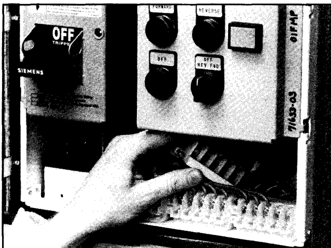
Figure 21B. Moving Terminal Blocks into the Wireway
