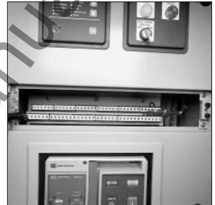
Secondary Control Terminals
