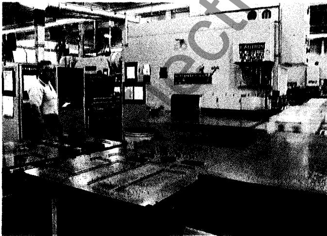
Numerically controlled machines meet the stringent requirements of GE switchgear design engineering.
