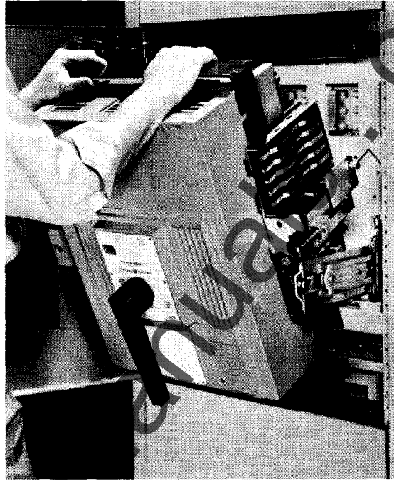
FIGURE 34. TILTING THE BREAKER
