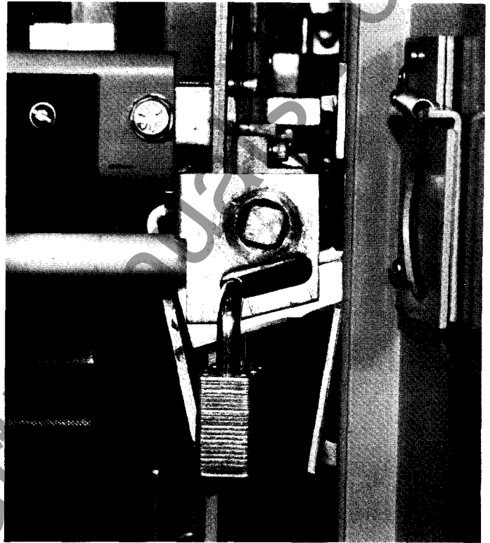
Fig. 7-7. Racking mechanism padlock device (AKR-75/100 breakers)
