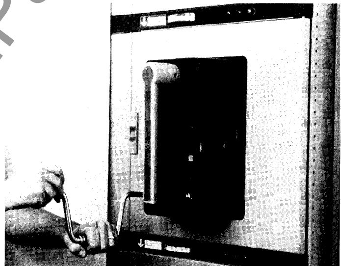
Fig. 7-1. AKD-8 switchgear circuit breaker in drawout position
