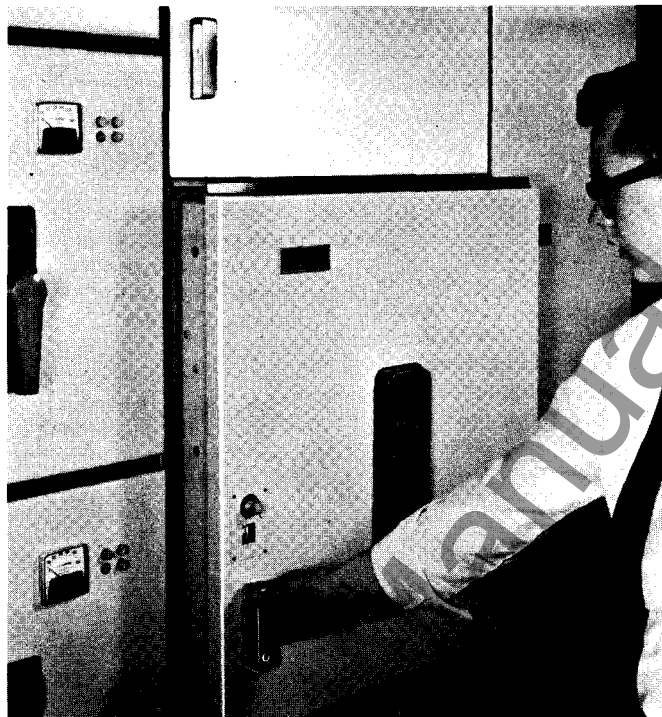
FIG. 16G (8035636) Push the breaker in completely and rotate the two track lock links. Close the door
