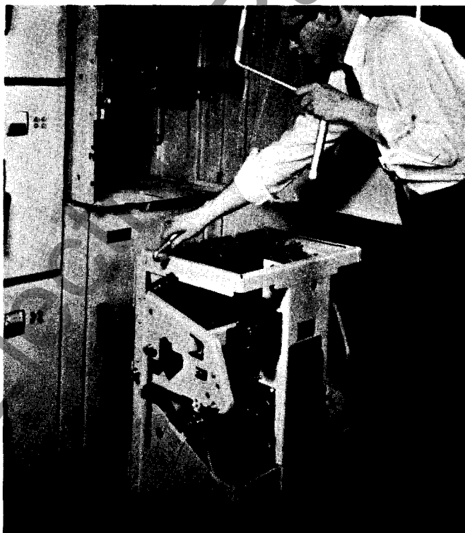
FIG. 16B (8035640) Let out Hoist Cable. Place hooks in slots.
