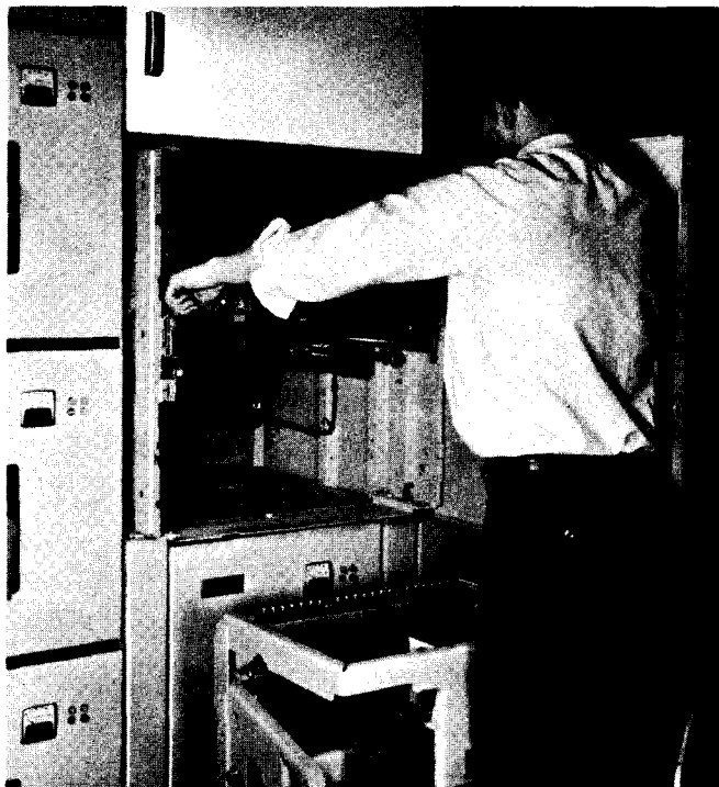
FIG. 16A (8035642) With innerhouse in DISCONNECTED position, open the compartment door. Rotate the two track lock links. Pull out right track completely.
