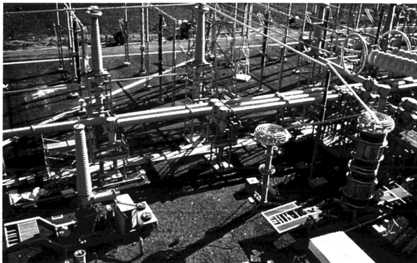
Dielectric tests on site, after erection
