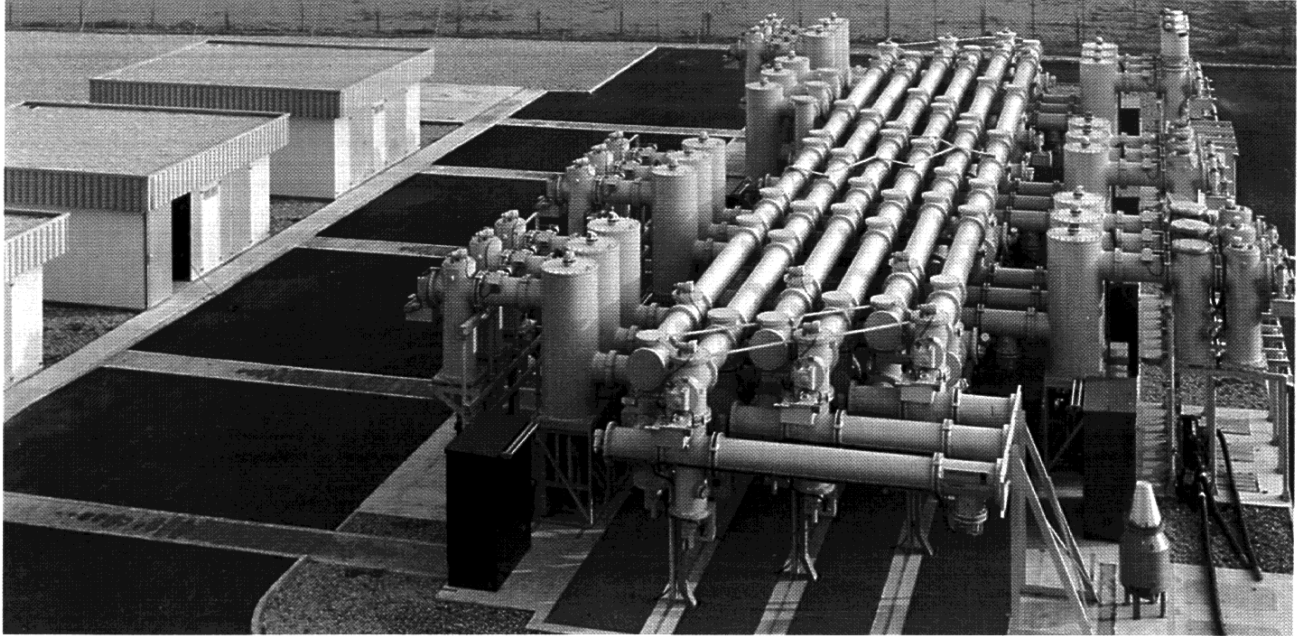
Section of a bay (double busbars and cable termination)
