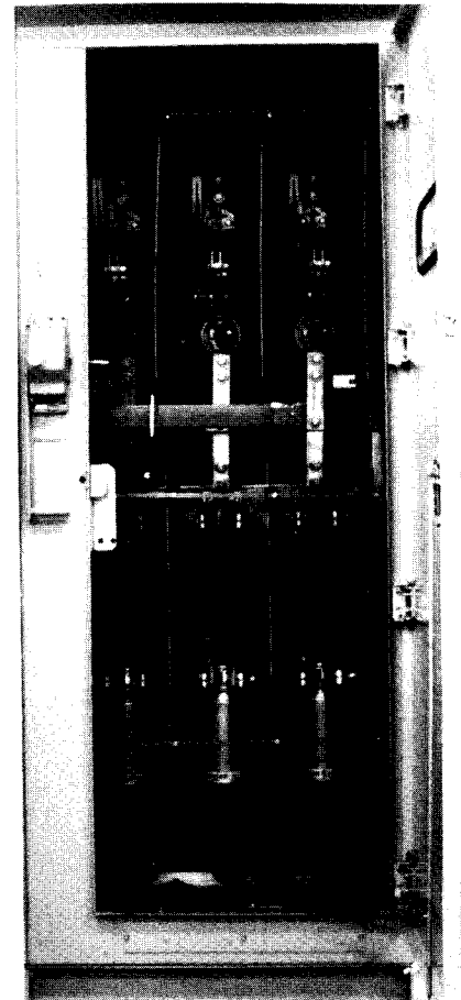
Figure 5. Unit Enclosure with Switch Module and Fuses Installed
