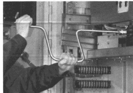
Levering Crank Operation (with door open for illustrative purposes)
