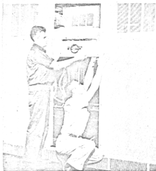
8. Assemble temperature panel (if furnished).
